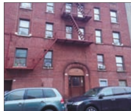
Photo by David Greene FDNY RESPONDED TO a reported ceiling collapse at 3469 Dekalb Avenue in Norwood on Feb. 7, 2025, pictured Sunday, Feb. 16, 2025, though the super of the building disputes the collapse.
